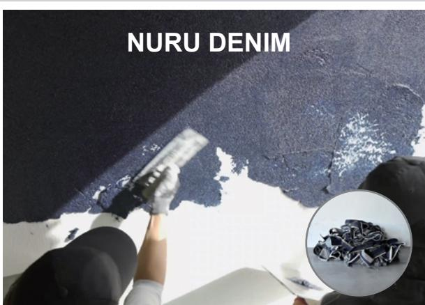
**NURU DENIM** is a plastering material upcycled from pulverized denim scraps, featuring a unique texture and excellent moisture controlling effects. It was developed as our initiative to address the growing issue of denim waste in Japan.
