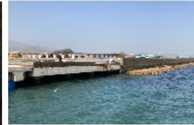
Under Port Piers
