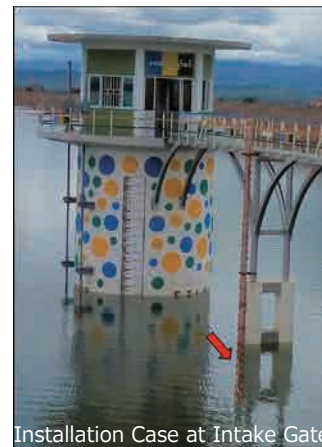
Installation Case at Intake Gate
