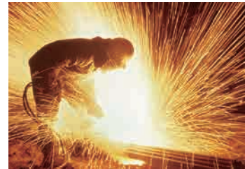
Gas fusion cutting
